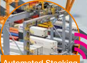
Automated Stacking Cranes (ASC) Trolley Travel Crane Travel
